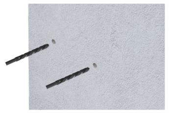
It is recommendable to make the blast-holes using a 6.5mm [1/4"] and a 8mm [5/16"] bits.
