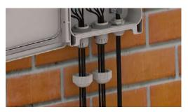
Fig. 16 Grommet rightly collocated.
