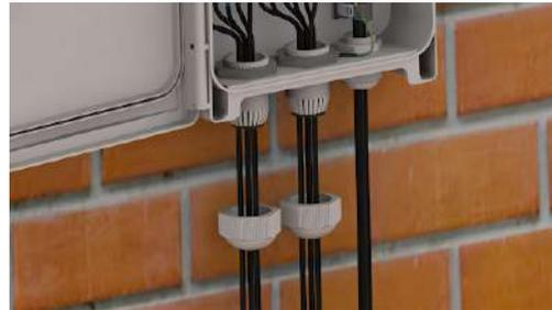
**Fig. 16** Grommet rightly collocated.
