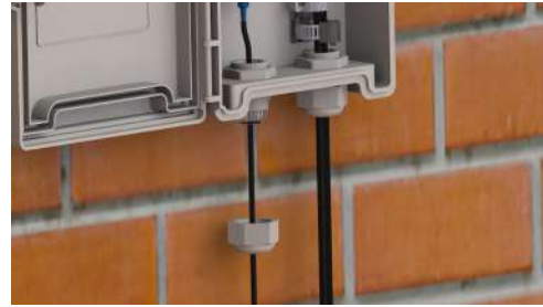
Fig. 13 Grommet rightly collocated.
