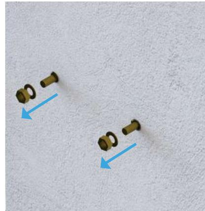
Align the multiport service terminal installation hole with the screw M8x1.0.
